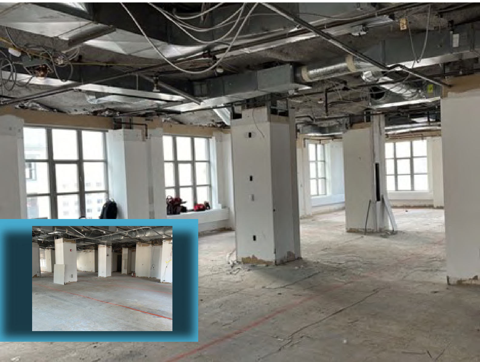
Before Photos; Jersey City, NJ
