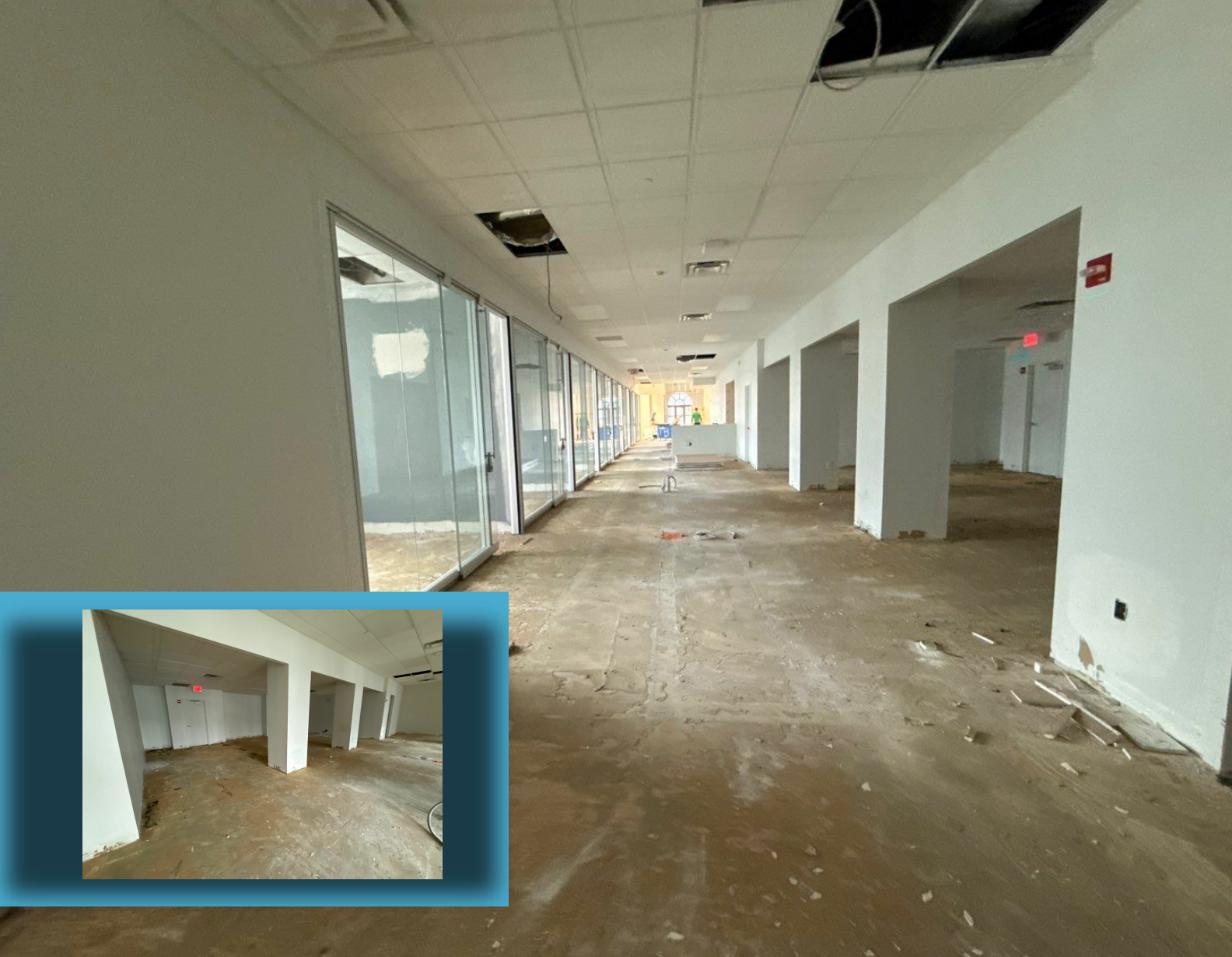
Before Photos; Jersey City, NJ
